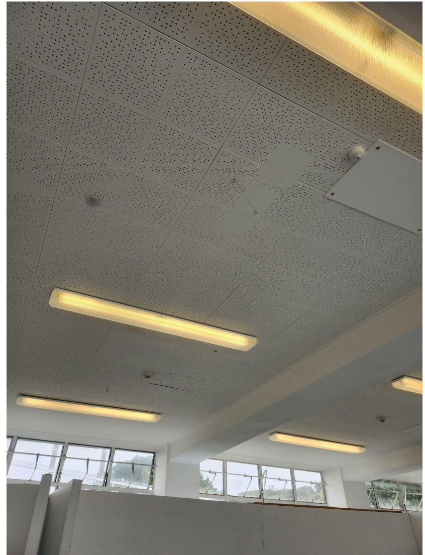
Fig. 77. Photograph of Block 2 Level D: ceiling, personal photograph by author, 20 January 2026
